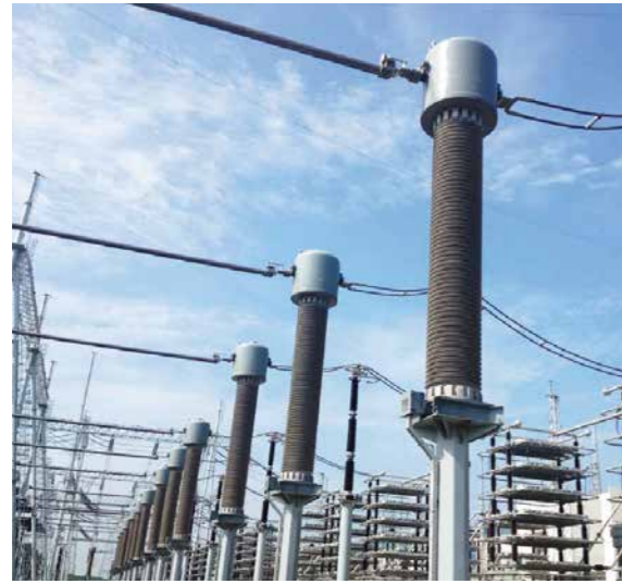
27.5kV-500kV Oil immersed inverted current transformer
