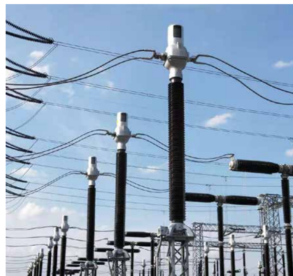
27.5kV-500kV Oil immersed inverted current transformer
